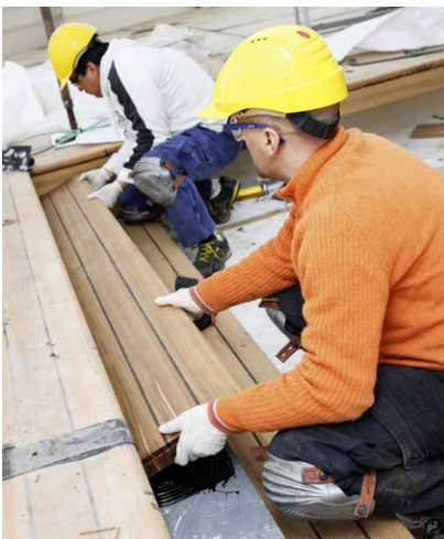
Fig. 13 Putting down the decking
