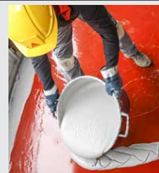
Fig. 7 Pouring the SikaTransfloor®-352 (SL/ST) to the floor
