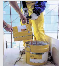
Fig. 6 Transferring the SikaTransfloor®-352 (SL/ST) to another container
