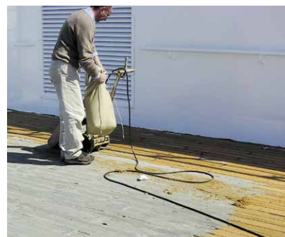
Fig. 20 Sanding the deck
