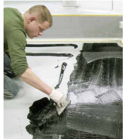
Fig. 55 Application of Sikaflex®-298
