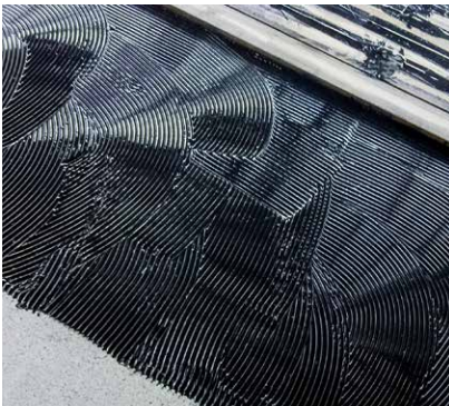
Fig. 12 Sikaflex®-298 applied with a comb spreader
