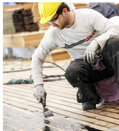
Fig. 19 Compressing Sikaflex®-290 DC PRO with a spatula
