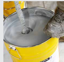
Fig. 5 Mixing SikaTransfloor®-352
