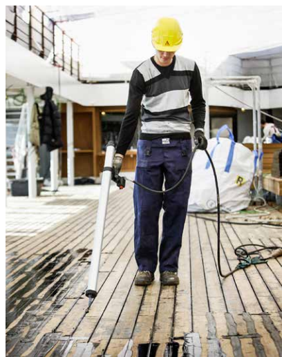
Fig. 17 Applying Sikaflex®-290 DC PRO
