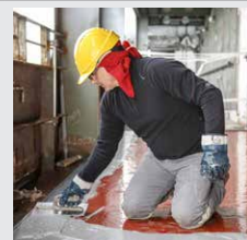
Fig. 8 Spreading the SikaTransfloor®-352 (SL/ST)
