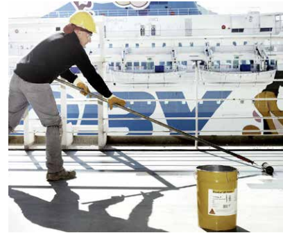
Fig. 3 Applying SikaCor® ZP Primer with a roller
